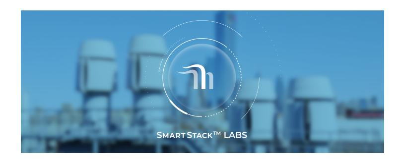
SmartStack™ is an active sensing system that constantly monitors the cleanliness of lab exhaust air and indexes the exit velocity of high plume fans according to the real-time level of contaminants in the lab exhaust air. This revolutionary approach ensures that dilution criteria are met and that concentrations of hazardous materials remain at safe levels, while maximizing energy savings.
